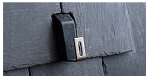
Figure 8: Solarflash on slate roof
